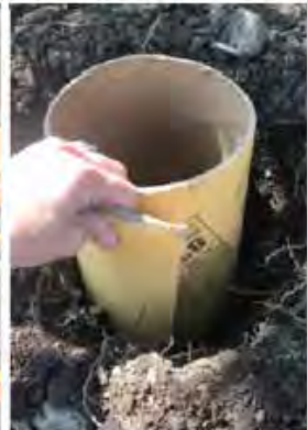
Cut down center of concrete form and place into hole.
