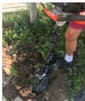
Post Hole - Use auger to dig initial hole.
