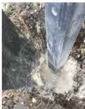
Aerate the cement
