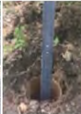
Set posts into center of post holes making sure to level/straighten.
