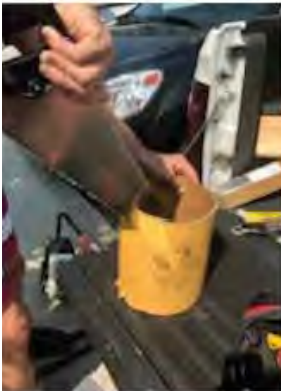
Cut two 1 foot concrete form cardboard tube sections.
