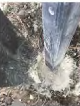
Aerate the cement
