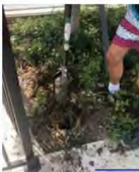
Post hole clean out shovel - Dig and clean both holes for 2 feet posts.
