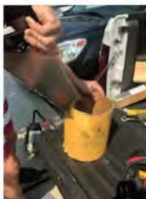
Cut two 1 foot concrete form cardboard tube sections.
