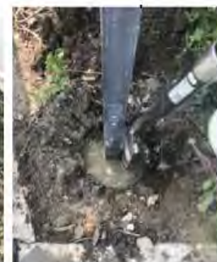
Aerate the cement again once water is poured
