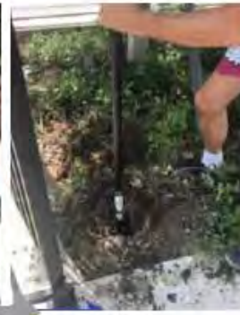
Post hole clean out shovel - Dig and clean both holes for 2 feet posts.
