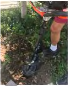
Post Hole - Use auger to dig initial hole.
