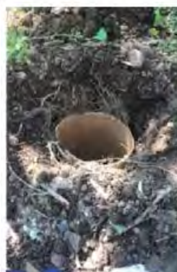
Post hole clean out shovel - Dig and clean both holes for 2 feet posts.
