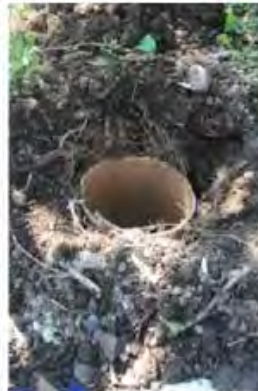
Cut down center of concrete form and place into hole.
